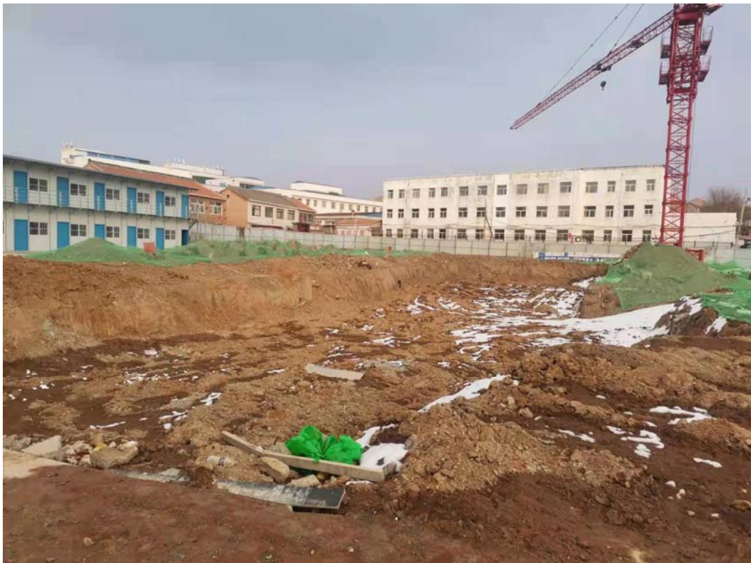
场内临建现状照片
